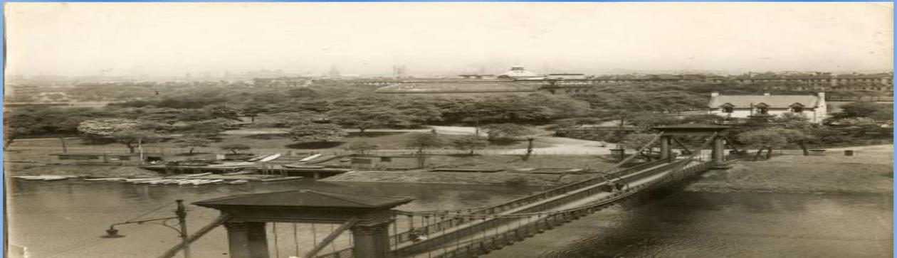
Our Tidal weir and pump Bridge keeps the water upstream at a regulated height---this was to enable factories to use the river water as a cooling system. The riverbank was built up using iron slag from the steel works—large stones laid carefully from the weir on the north bank to Tollcross and from the weir to Rutherglen on the south bank. This stone rebaiting and the fact that we do not get a low tide upstream of the weir--keeps the banking in place and stops it subsiding into the river
